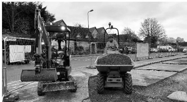
Charger installation work at New St car park
