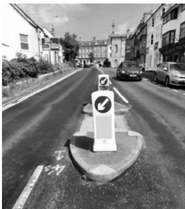
Improved signage & safety items should make pedestrians safer
