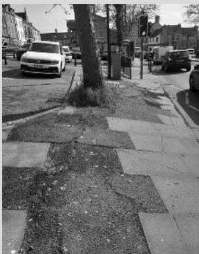
OCC – ‘Levelling up’ needed! Bodged tarmac job. Why not a raised green bed?
